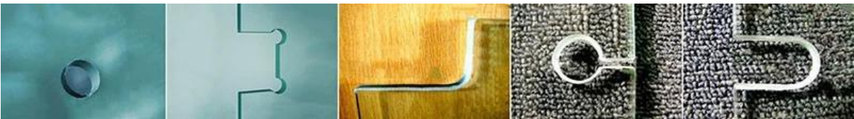
Breakage of toughened laminated glass:
