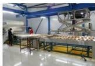
合片室设备 Clean Room Equipment
