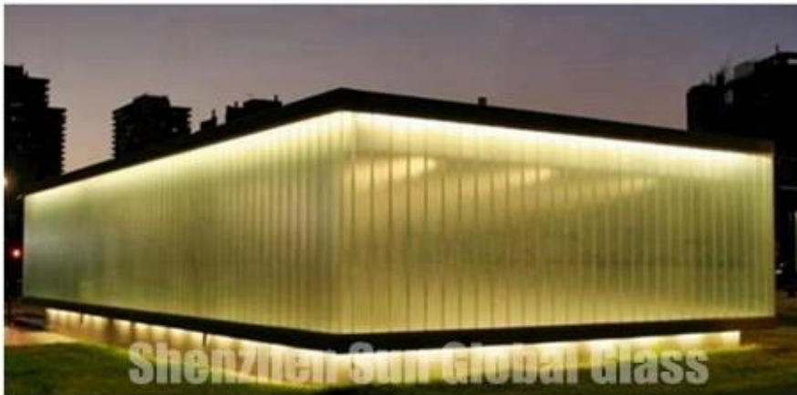
Picture of 7mm low iron U profiled glass:
