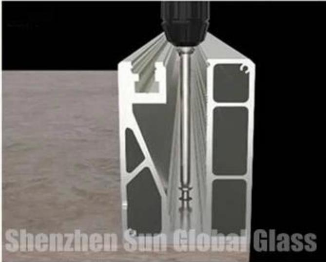
**screw the aluminum groove to the floor
