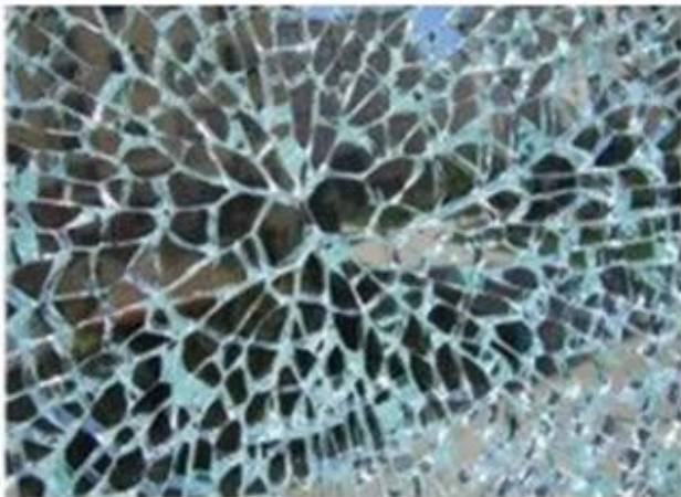
tempered glass broken with normal external force cubical debris won't fall down
