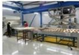
合片室设备 Clean Room Equipment
